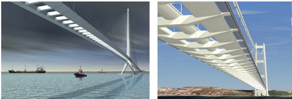
Fig. 4 - Multiple-box decks examples: Chongming bridge in Shanghai, cable-stayed bridge with central-span length equal to 730 m, on the left, and Messina bridge '92, in Italy, suspension bridge with central-span length equal to 3.300 m, on the right.
