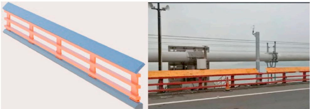
Fig. 2 - Installation of spoiler on Humen Bridge.
