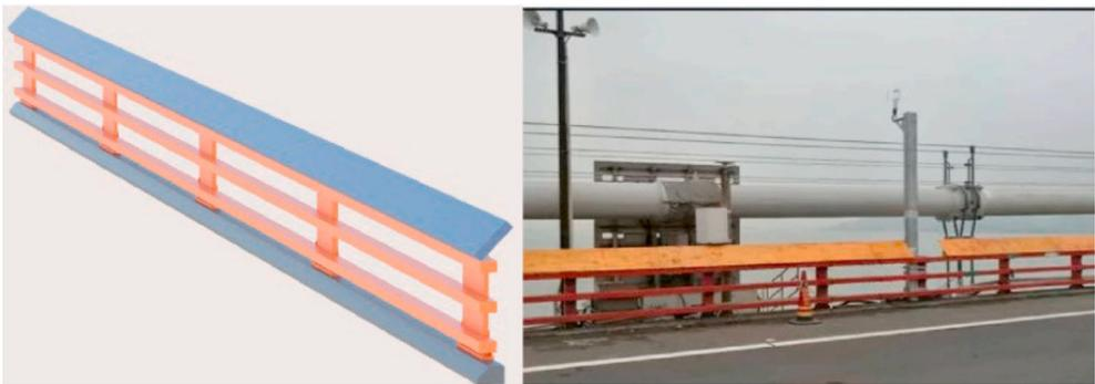
Fig. 2 - Installation of spoiler on Humen Bridge.
